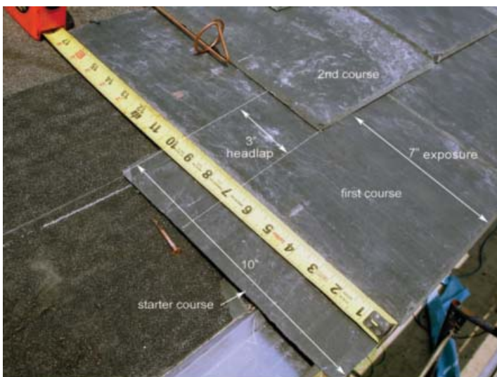
Figure 7: Common mistakes made when installing starter courses include orienting the starter slate face side up, installing no cant, inadequate headlap, and insufficient side-laps. [Photo by Joseph Jenkins]
