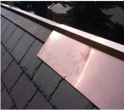
Figure 3: The old copper ridge was removed and wider, new copper ridge was installed, leaving a generous 5" headlap on the second course of slates where there was no headlap before. [Photos by Chris Short]
