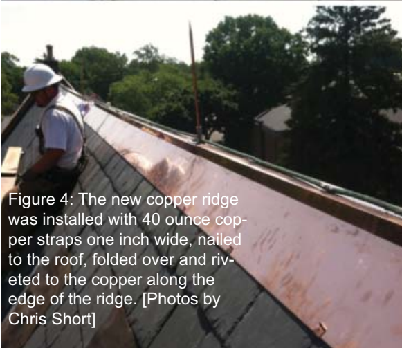
Figure 3: The old copper ridge was removed and wider, new copper ridge was installed, leaving a generous 5" headlap on the second course of slates where there was no headlap before. [Photos by Chris Short]
